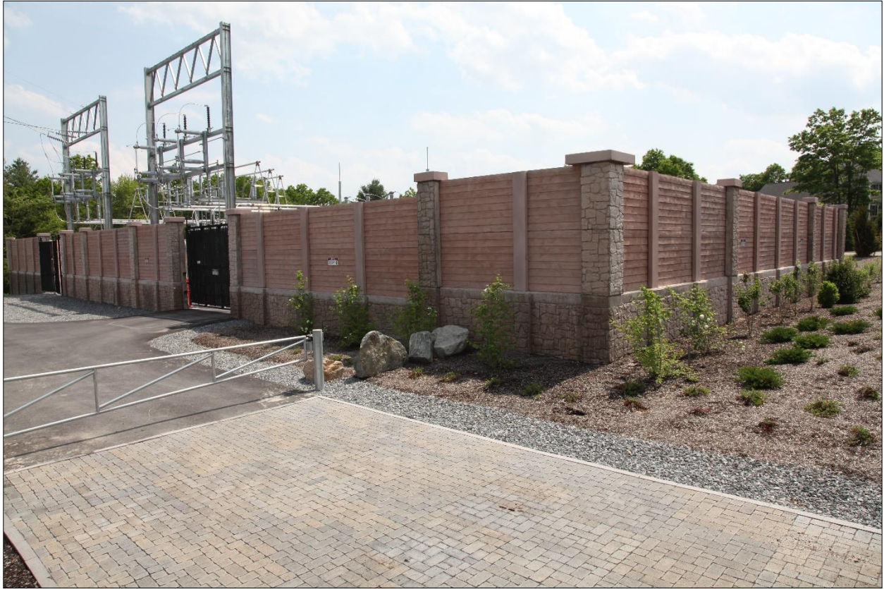
Figure 3: Example solid substation fencing 3
