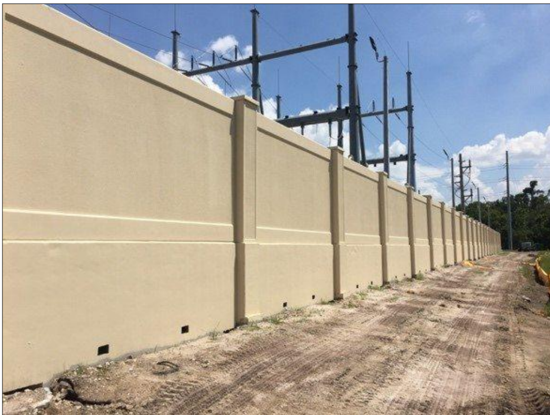
Figure 2: Example solid substation fencing 2
