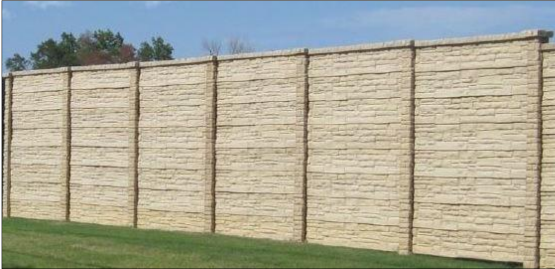
Figure 1: Example solid substation fencing 1
