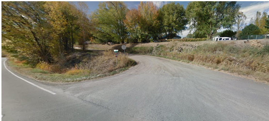
Figure 5: 3500 Road at SH 133
